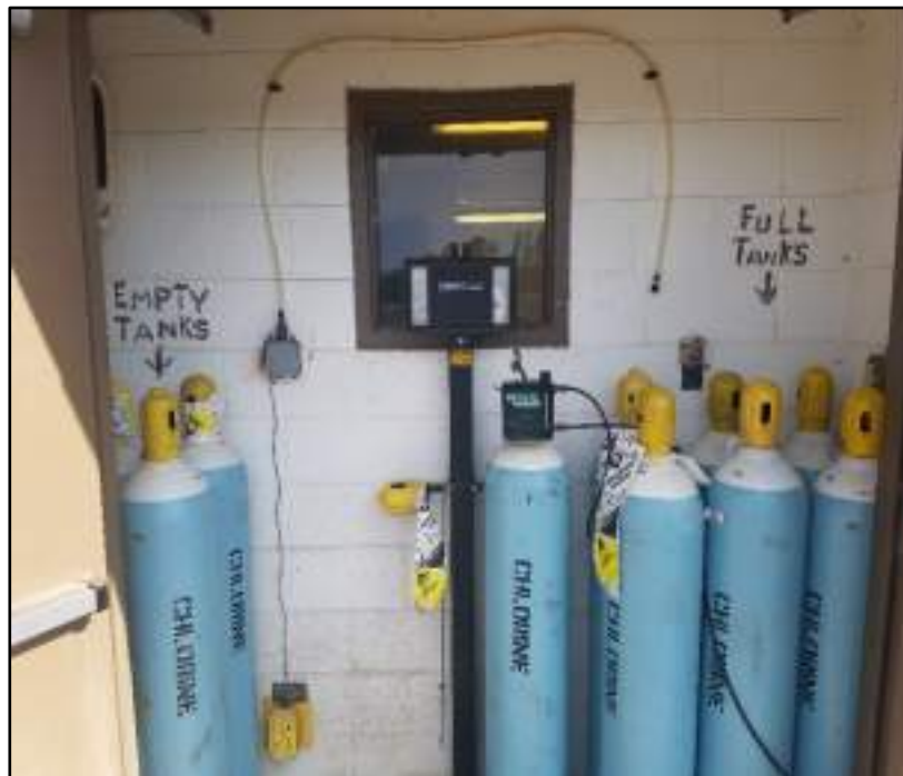
FIGURE 4-13: GAS CHLORINE SYSTEM
