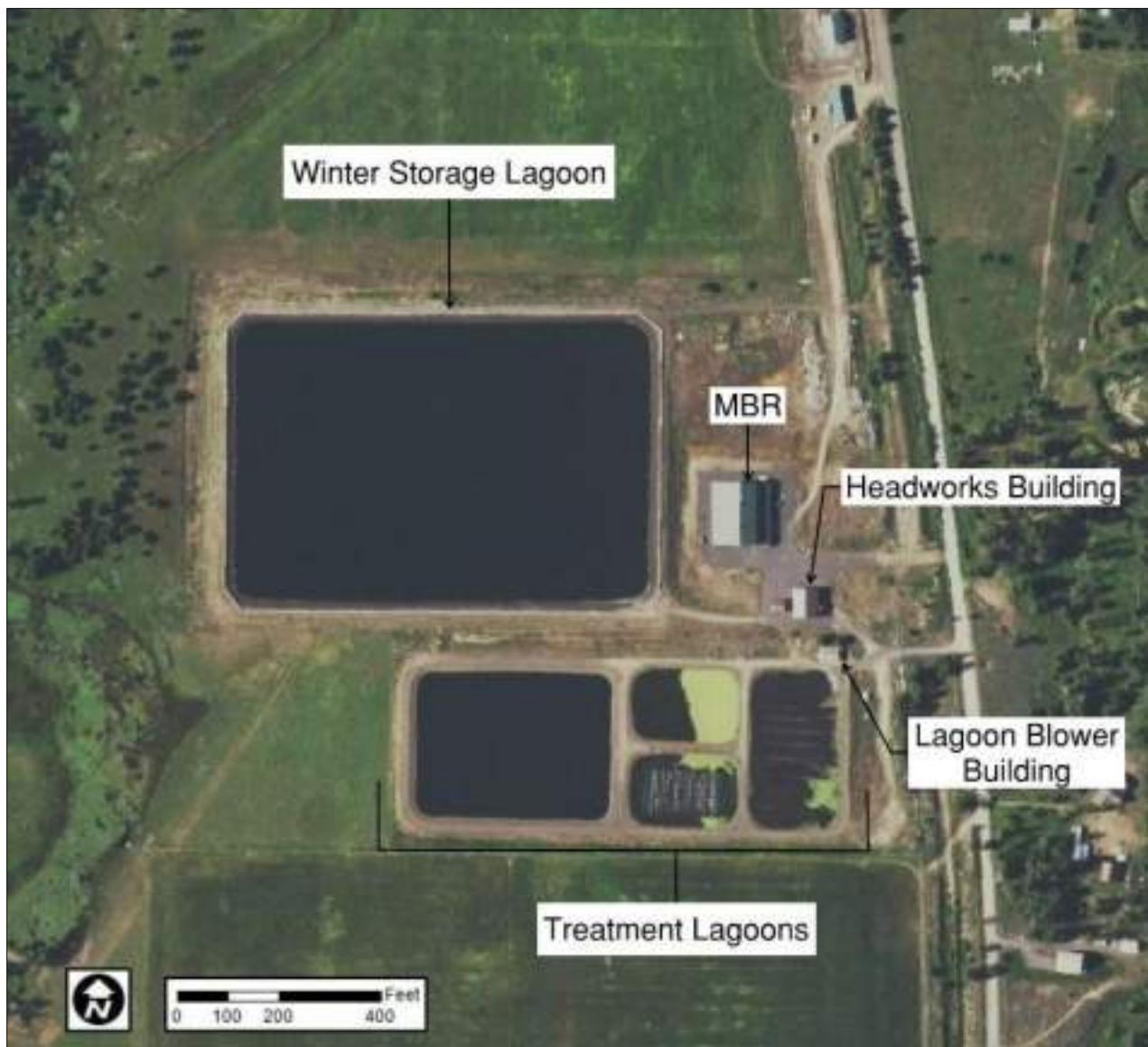
FIGURE 4-1: WWTP AERIAL VIEW
