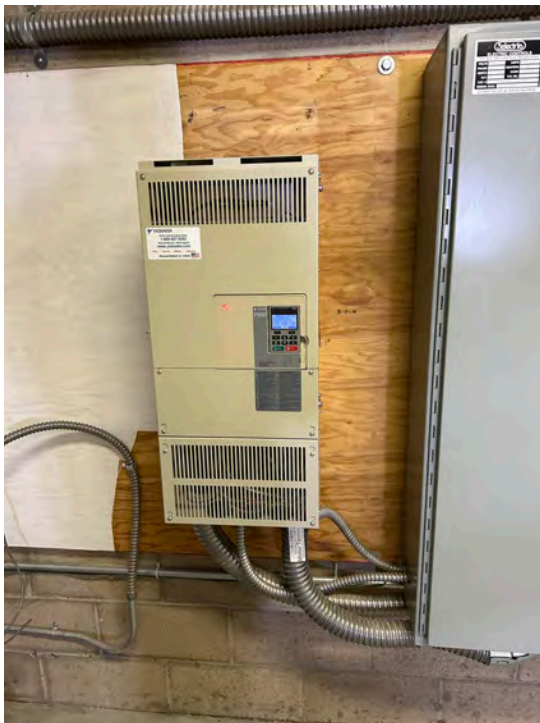
Photograph 6: Well #2 VFD
