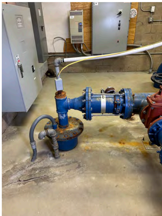
Photograph 1: Well #1 wellhead
