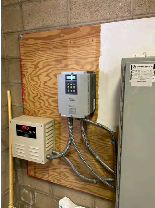
Photograph 7: Well #1 VFD
