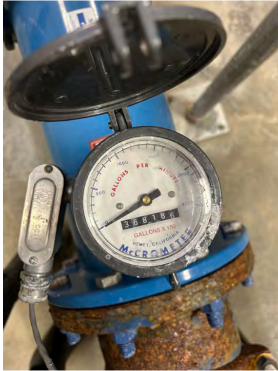
Photograph 9: Flow meter - 36818600 gallons
