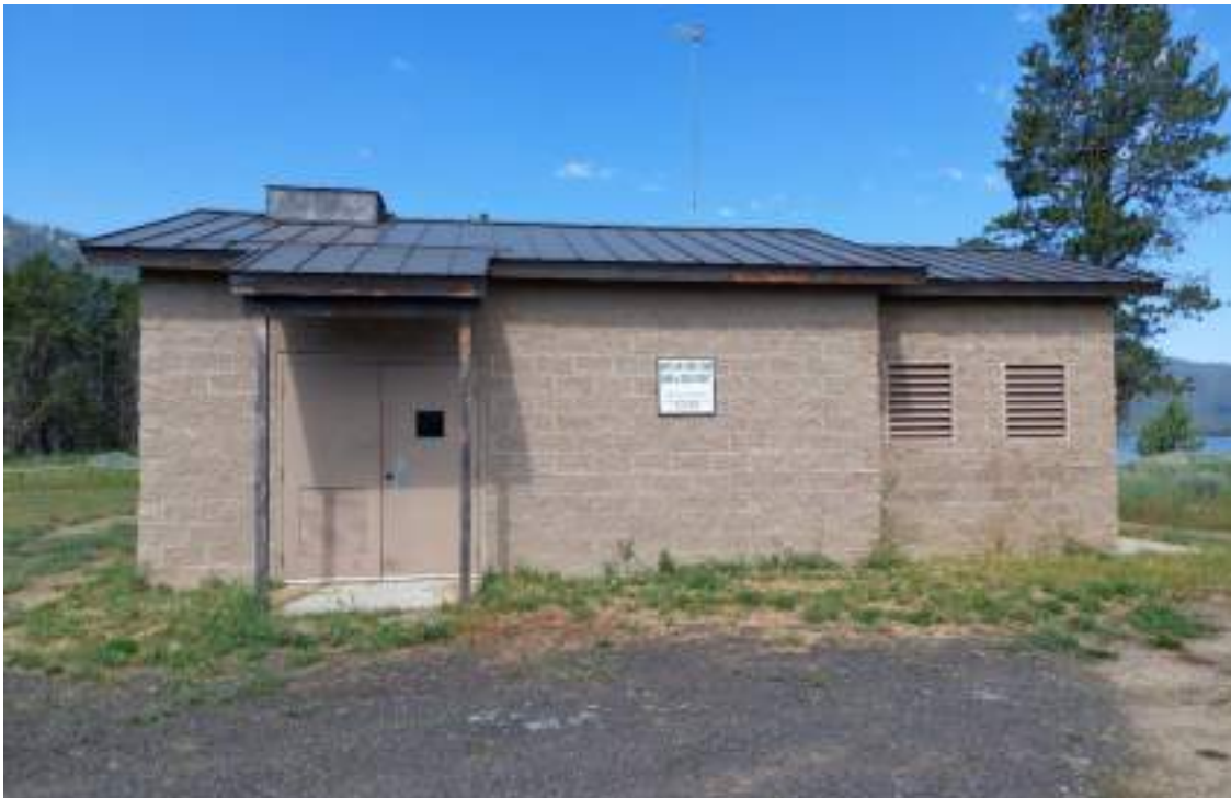
FIGURE 3-10: HAWKS BAY WELL SITE
